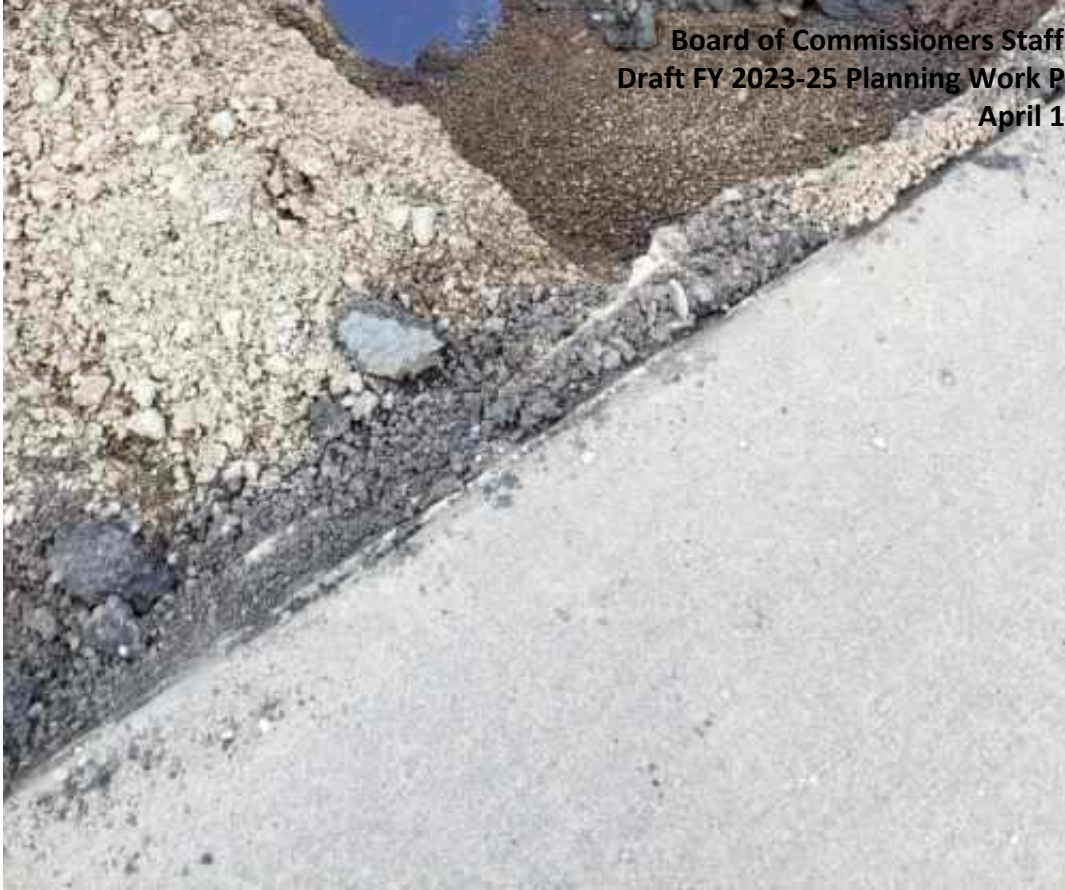
Fuel mixed with groundwater at a gasoline leak at Highway 99 and Main Street in Monmouth in April 2021. [Department of Environmental Quality]
