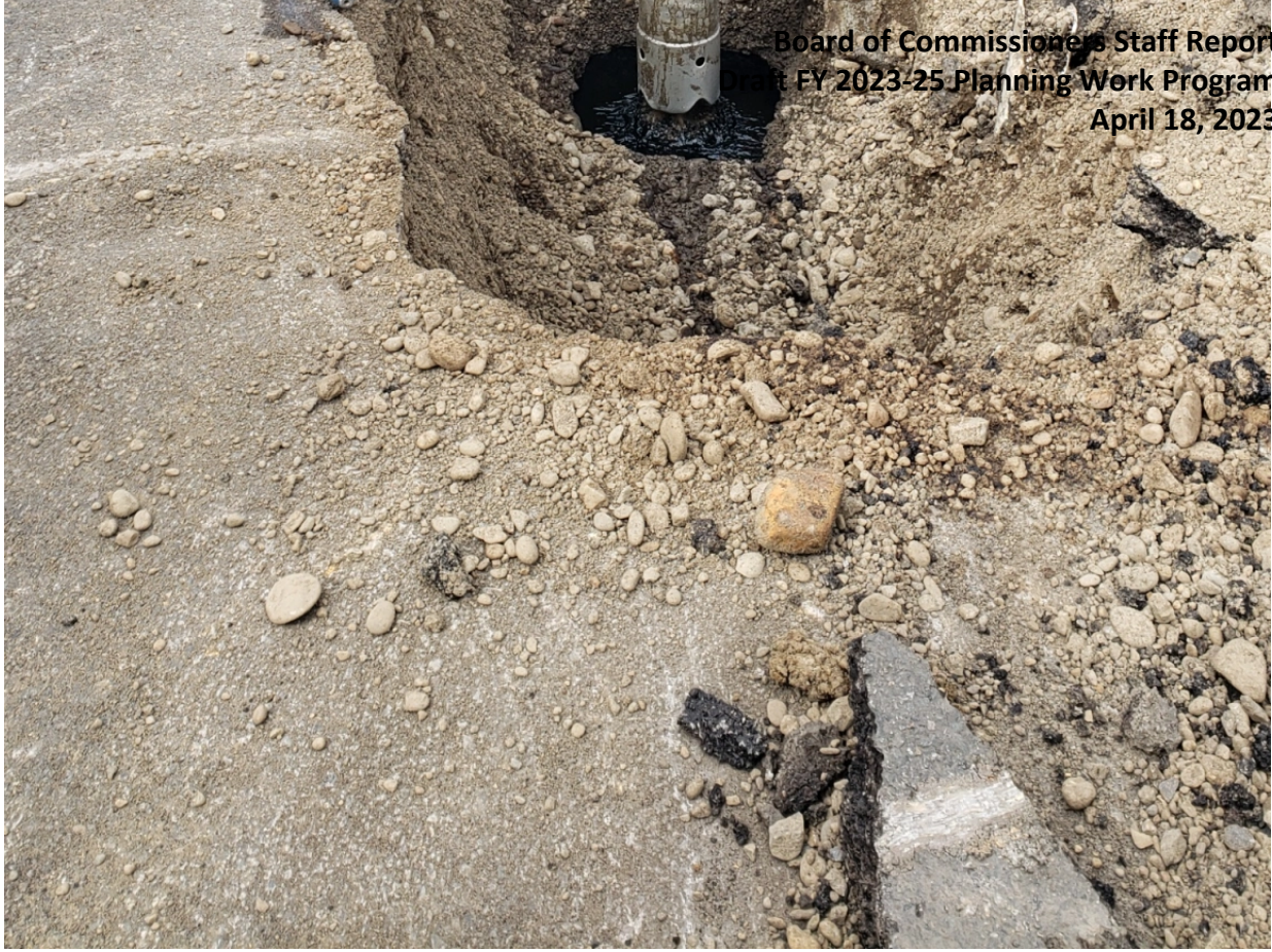
Removing gasoline that spilled from an underground storage tank at Highway 99 and Main Street in Monmouth in April 2021. [Department of Environmental Quality]
